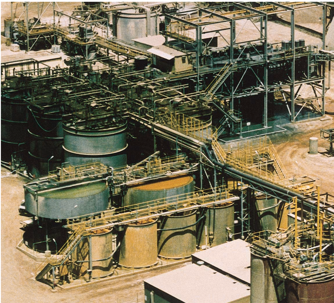
The BIOX ® plant at Wiluna Gold Mine, Western Australia, whose reserves are mostly refractory sulphides.
