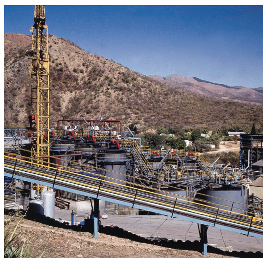
The Fairview BIOX ® Plant in Mpumalanga province, South Africa, which currently treats 55 tonnes of concentrate a day.
