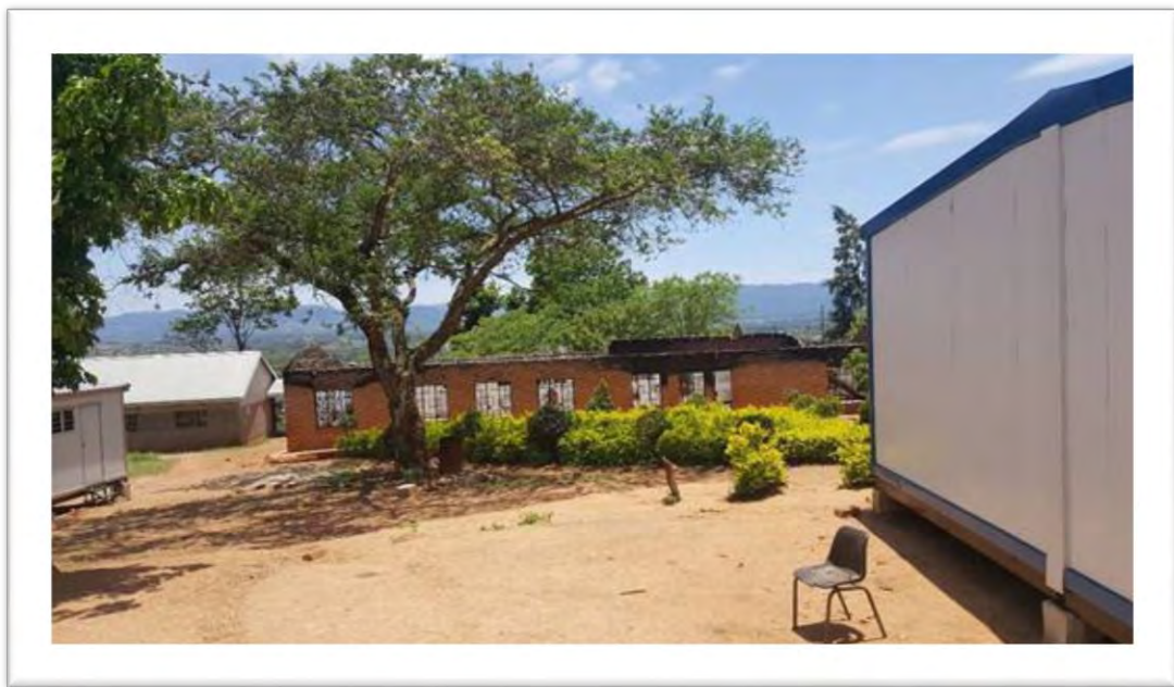
Figure 2.2: Burnt classroom block and planted prefab
